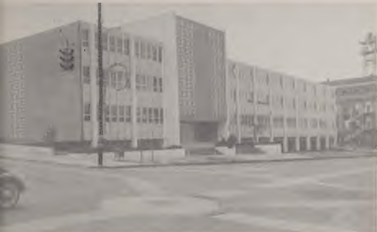
The County Court House at SW corner of Lawrence and Washington Street in 1962.
